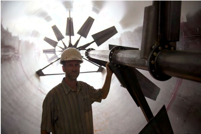
John Edel, founder of Bubbly Dynamics, inside the full-scale anaerobic digester.
